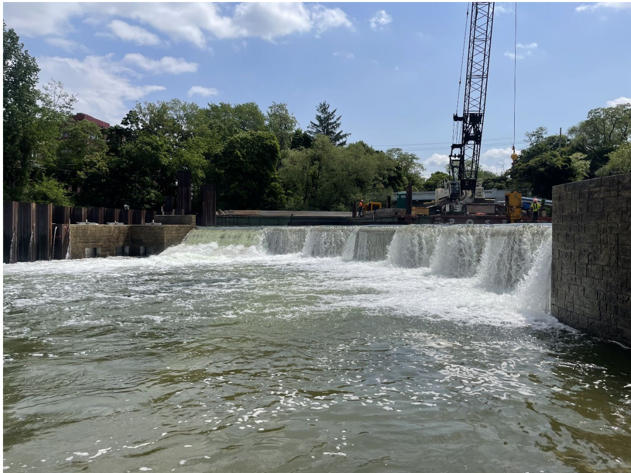
Figure 2. Rerouting of the Boardman/Ottaway River to pass over the new arc-labyrinth and low-flow weirs. Switching of flow from the old Union Street Dam to the new structures occurred on June 16, 2025.
